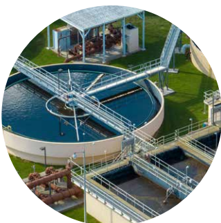
Future-Ready Water Systems and Infrastructure
